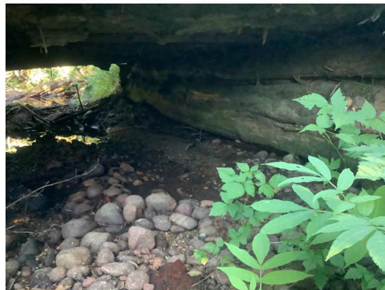
Left Bank Abutment when facing downstream
