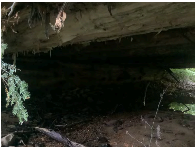
Right Bank Abutment when facing downstream
